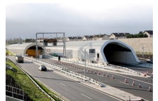
Dublin Port Tunnel
